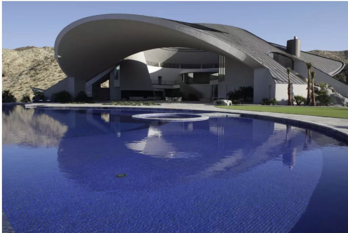
Architect John Lautner had the Bob Hope house built into a hillside overlooking Palm Springs. (Myung J. Chun / Los Angeles Times)
